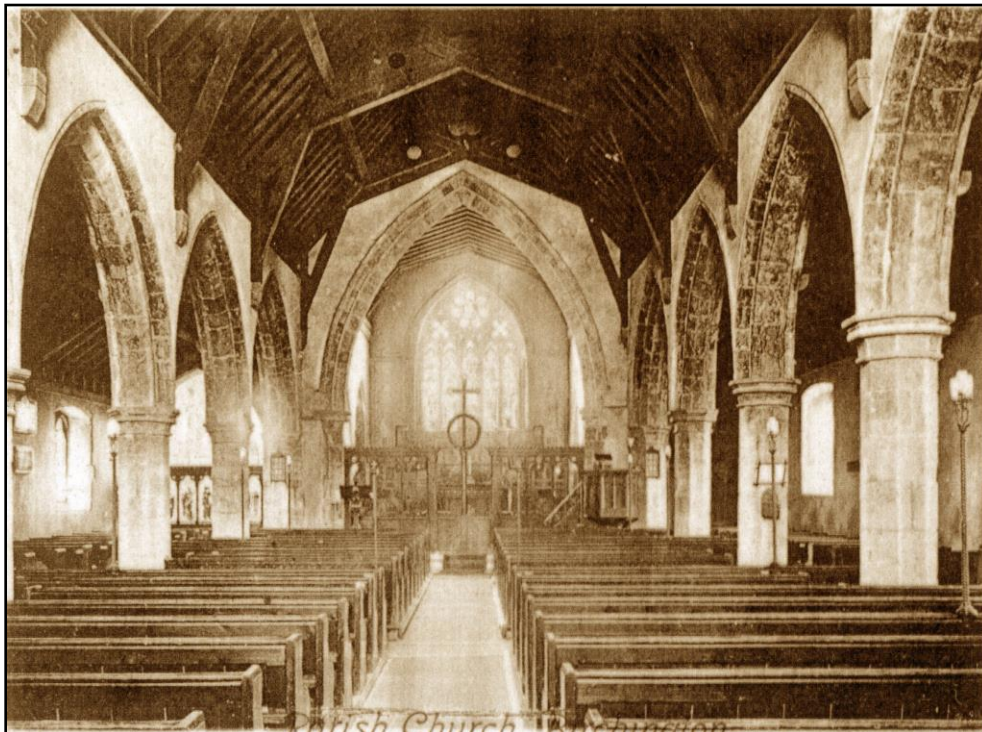
All Saints Church in 1926, showing the gas standards
