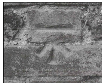
Benchmark in Reculver Avenue
