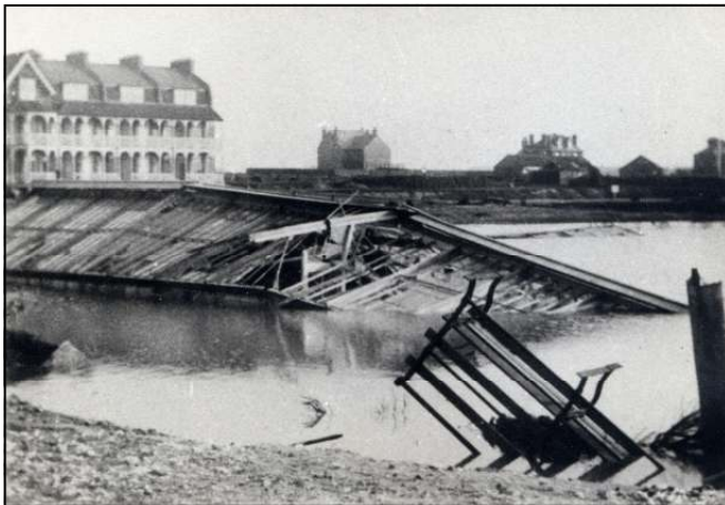
Storm damaged Exhibition building in the Minnis Bay Dip, c. 1897
