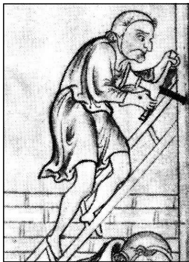
Stonemason working on a socket
