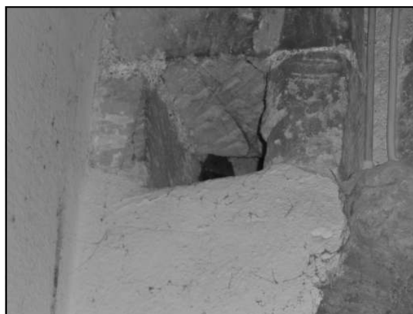
Beam hole in South West Aisle
